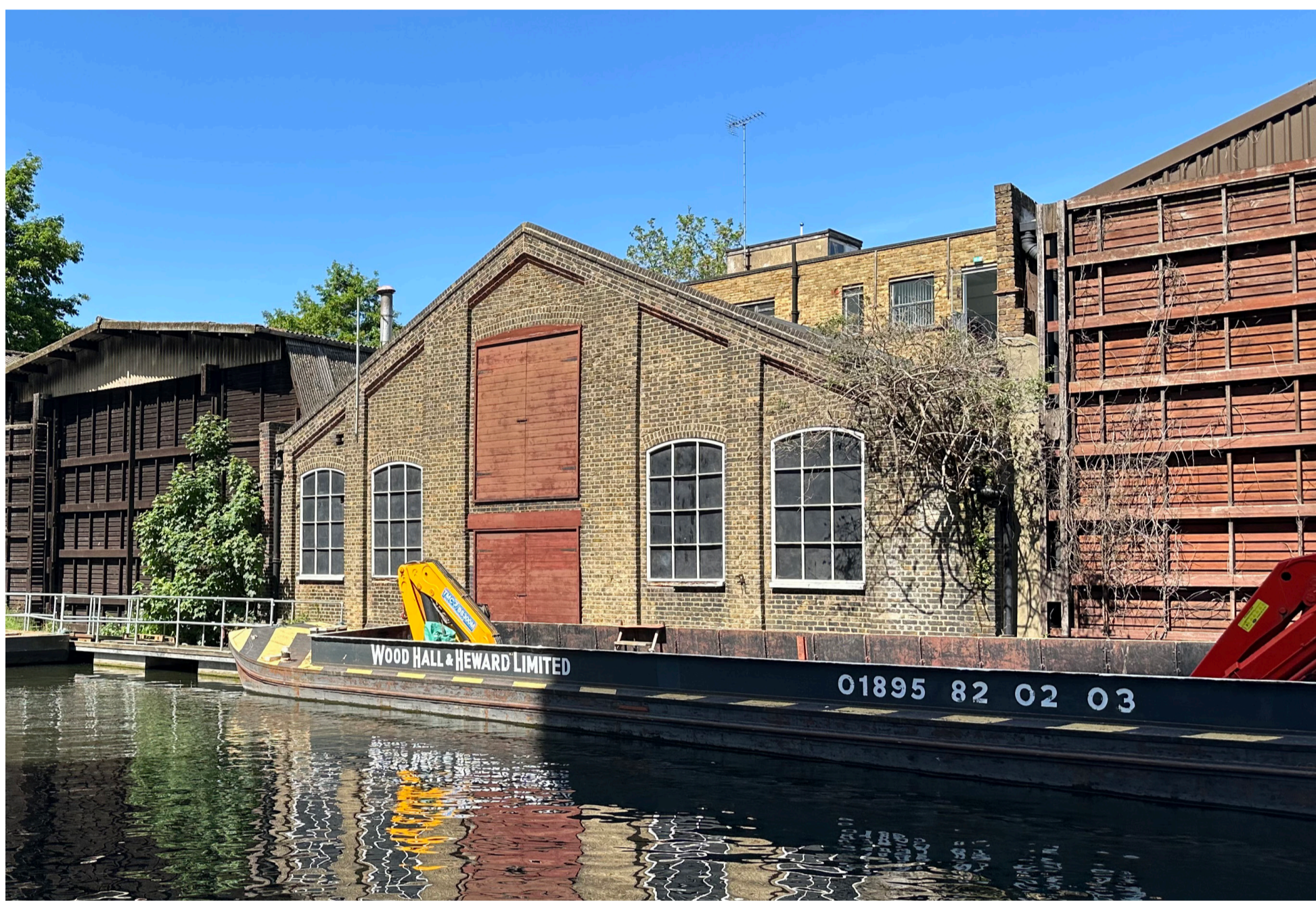
Gable in current arrangement
