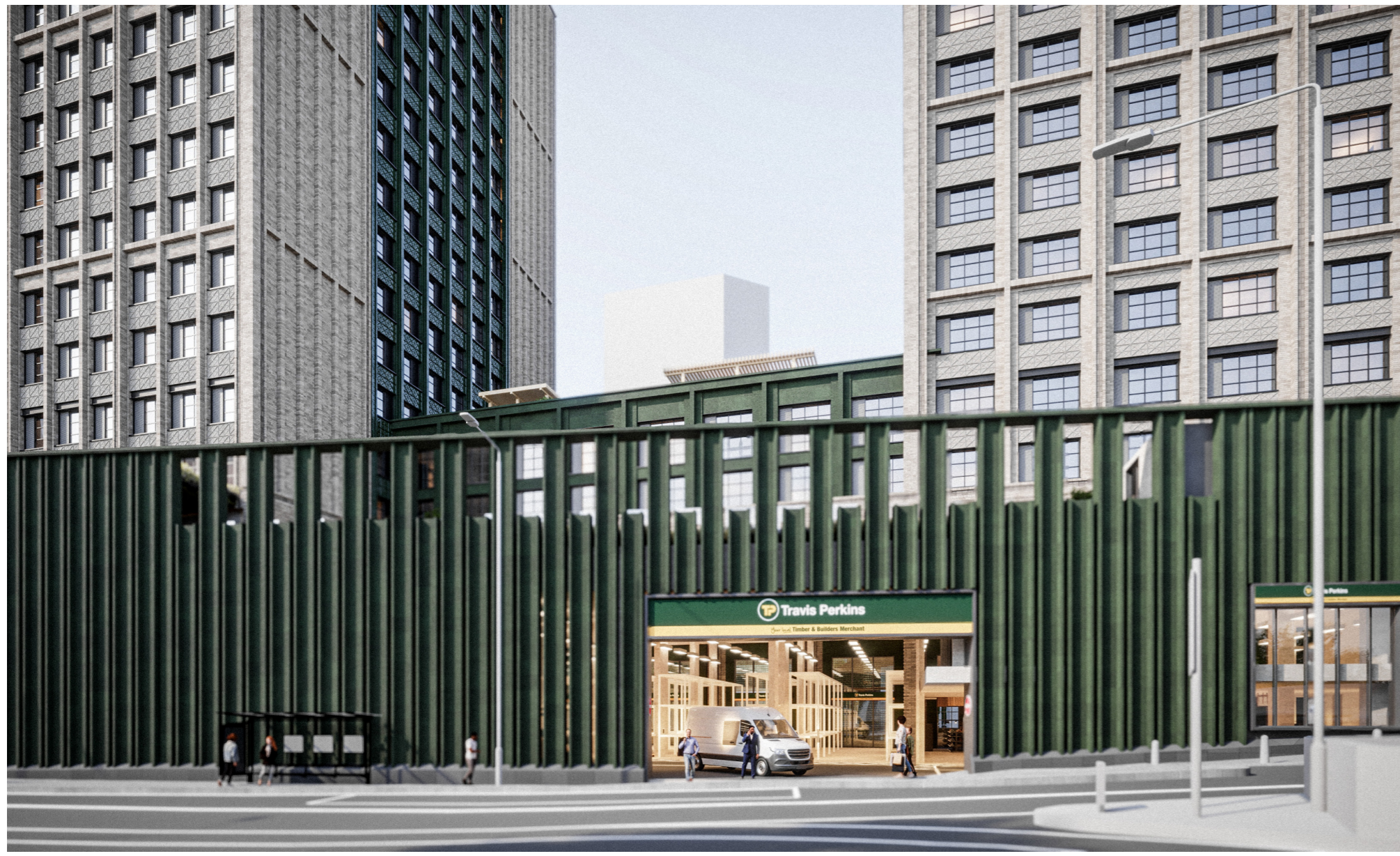
View of exit from Travis Perkins yard onto Harrow Road
